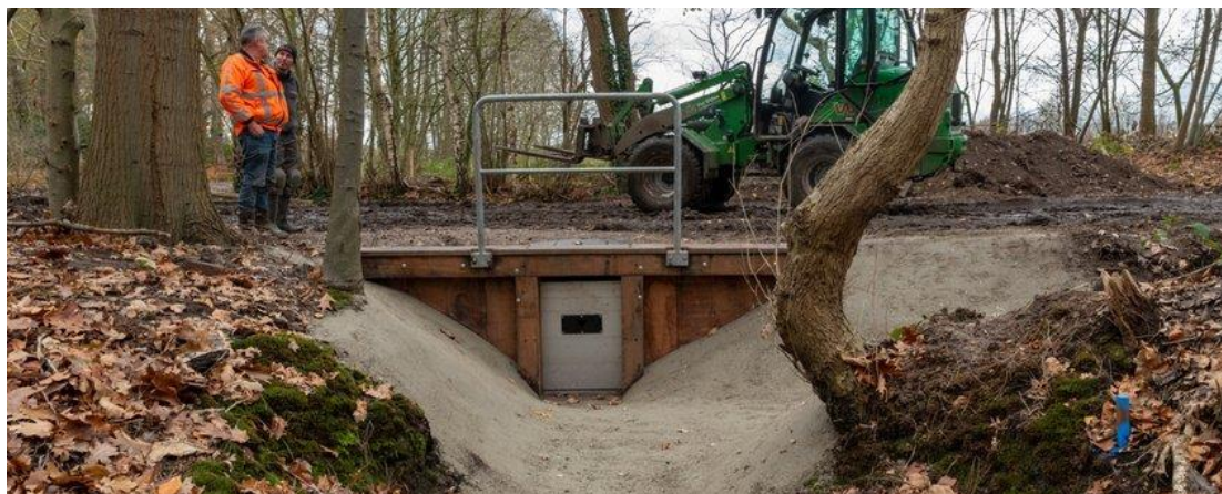
Figuur 36: Regelbare knijpstuw Ulvenhouts bos (Nederland) (bron: www.naturetoday.com )
